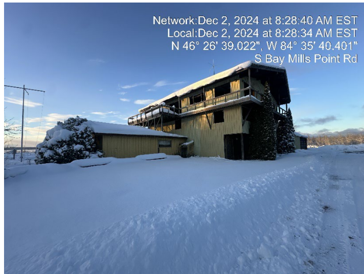
3-Story, 6,550-SF Commercial/ Residential Building with attached 3,520- SF Garage/ Workshop
